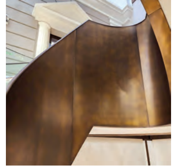
Detail of interior curved bronze cladding
