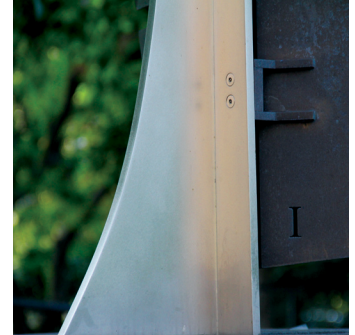
Detail of the Stainless Steel Mast
