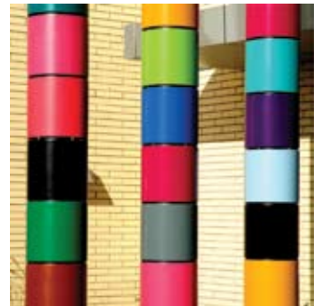
Detail of three (3) of the 24' cylinders
