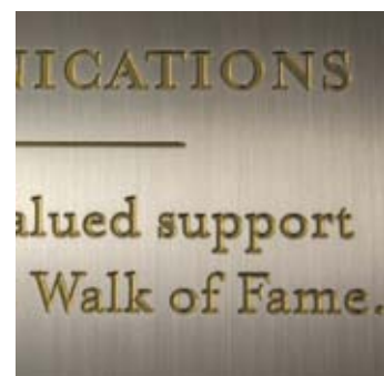
Detail of the etched and infilled gold text
