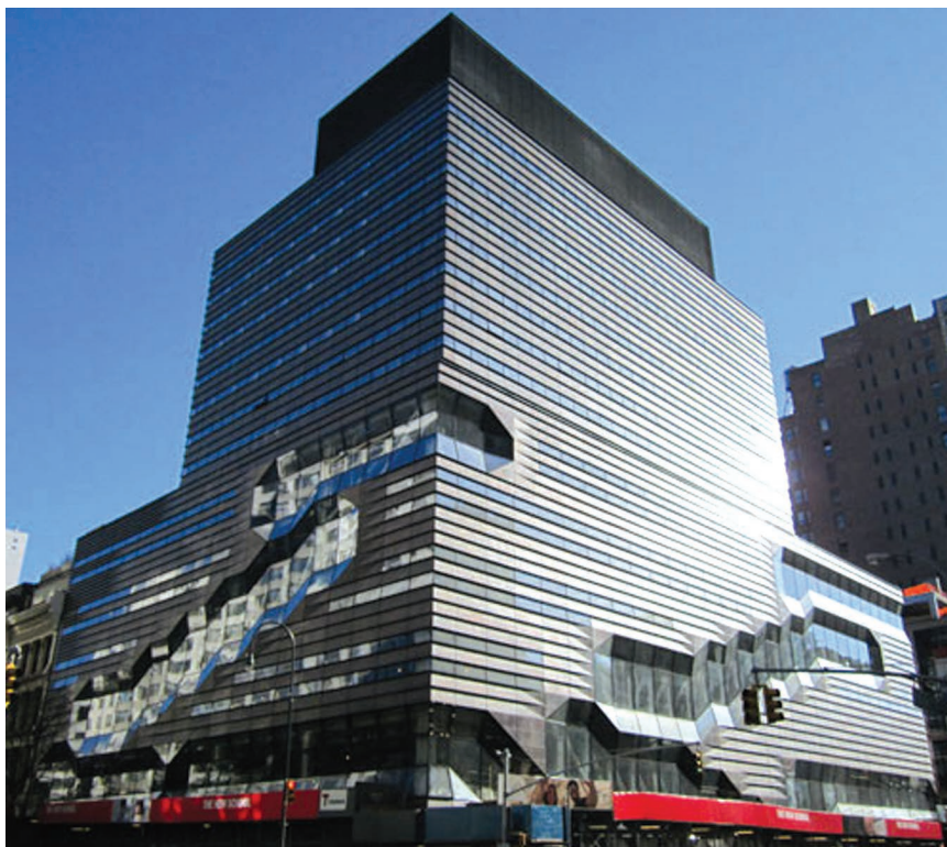
The New School at 65-5th avenue with completed cladding of the building envelope.
