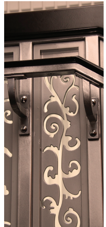
Detail of panel, railing and fasteners.
