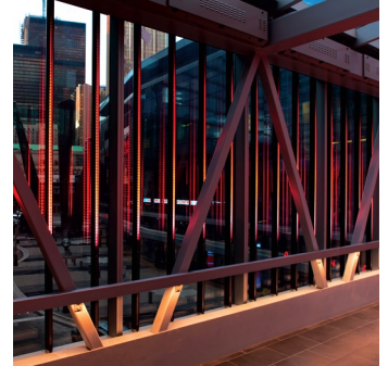
An interior view of the bridge
