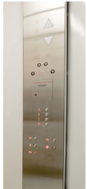
Stainless steel control operating panel (COP)
