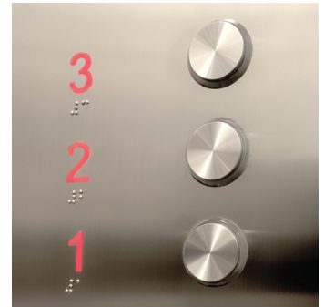
Detail of the COP with braille embossing
