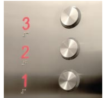
Detail of the COP with braille embossing
