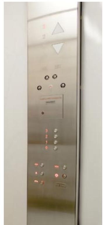
Stainless steel control operating panel (COP)
