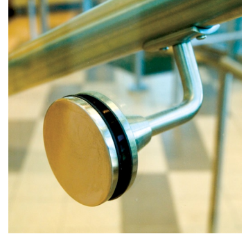
Railing support detail
