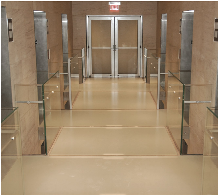
Glass bridge services elevator entrances
