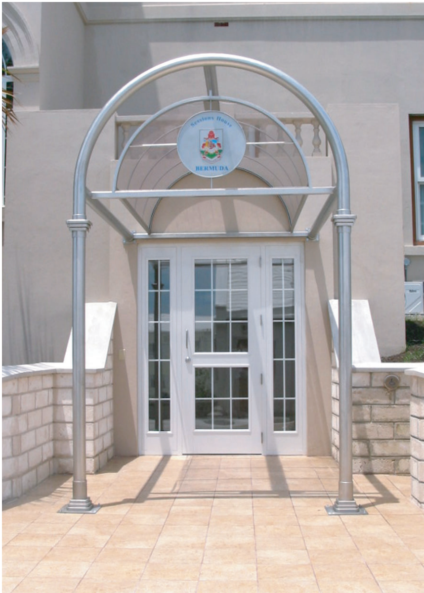
Stainless steel canopy with rolled 3/8" thick Lexan glazing (on location)
