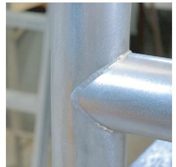
Strong structural weld
