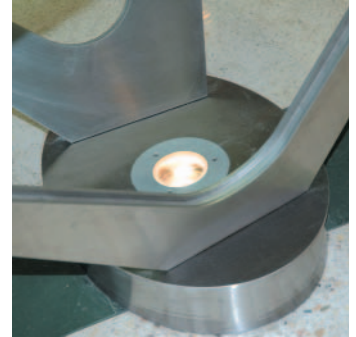
Recessed halogen flood light
