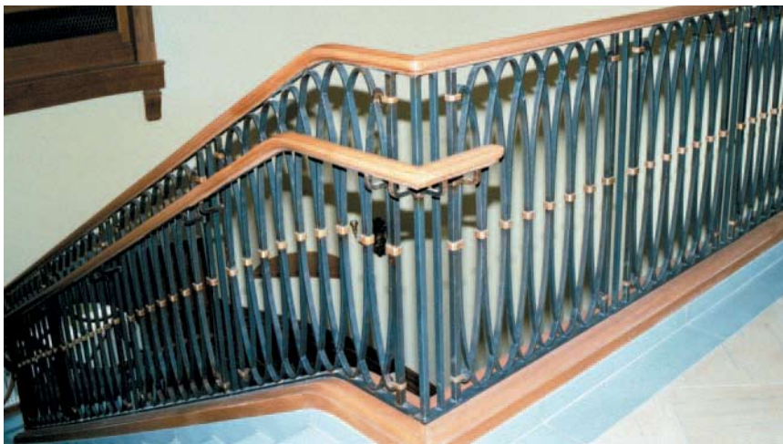
Guardrail and handrail
