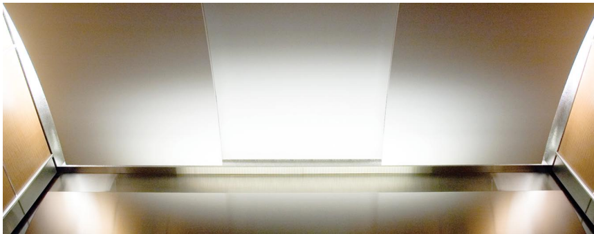
Painted aluminum ceiling carries the undulating design from the lobby into the elevator cabs
