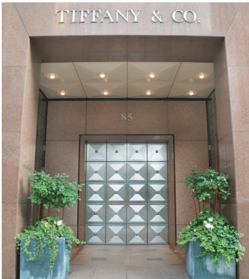
Entrance with security doors closed
