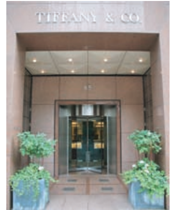
Entrance with security doors open
